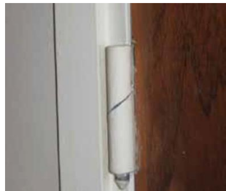
Figure 5 Rising Butt Hinge
