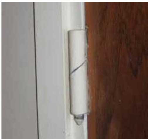
Figure 12 Rising butt hinge
